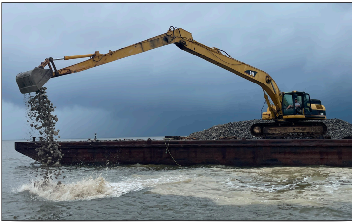
Crane on barge deploying rock at the Lynn Dent Boykin Reef.
