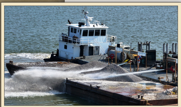
High pressure water cannons disperse the limestone oyster cultch material onto the Cedar Point Beach project site. The goal: one inch thickness across the 77-acre project site.
