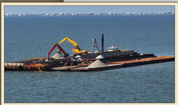
Cranes offload limestone cultch material from the deep hopper barges onto flat barges capable of entering the shallow waters at the Cedar Point Beach Project site.
