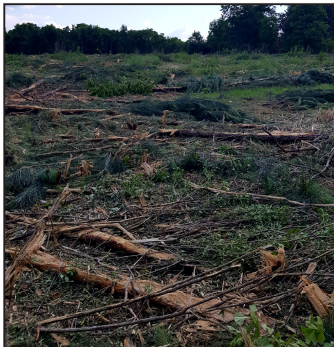
Mulching was utilized as the initial site prep treatment.
